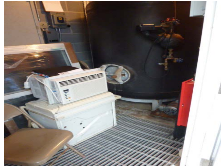
Expansion tank in mechanical closet at Community Center with 2,000 gallon domestic water storagetank in pit below grate.
