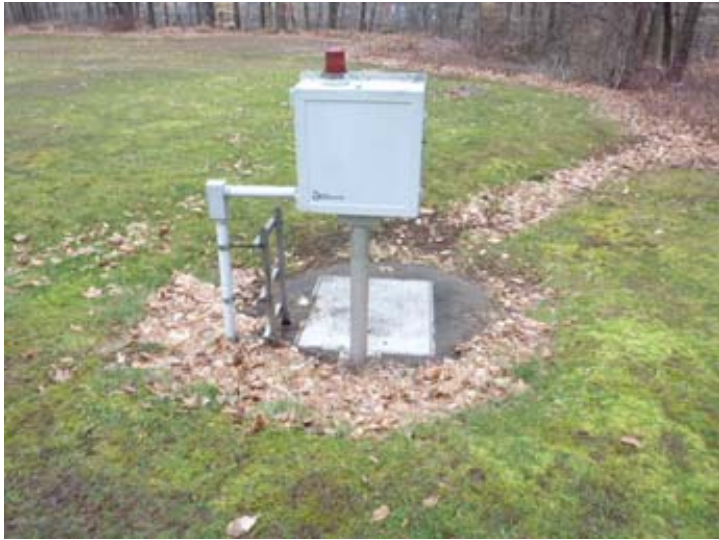
Sewage pumping station at opposite end of site from leaching fields.
