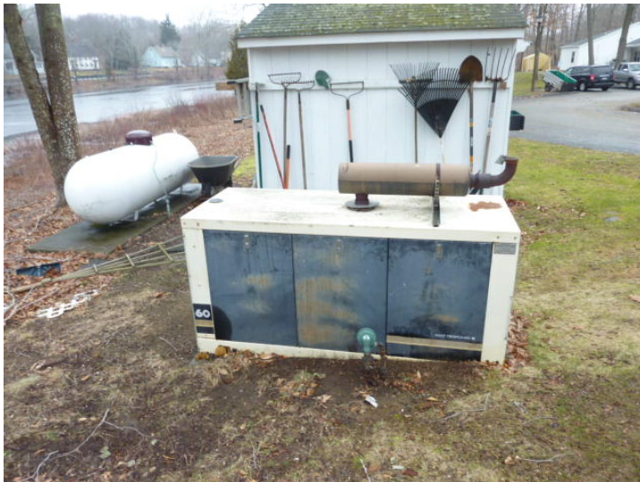
Gas-fired emergency generator behind Community Building.
