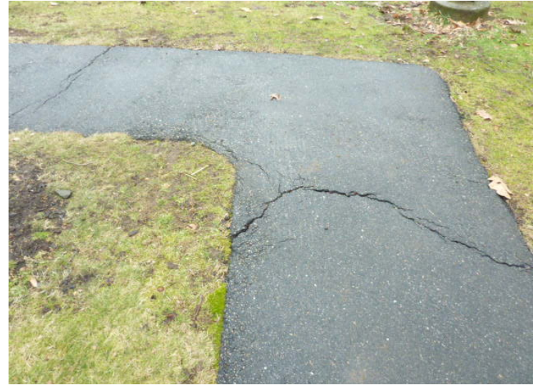
Typical asphalt walk failure.
